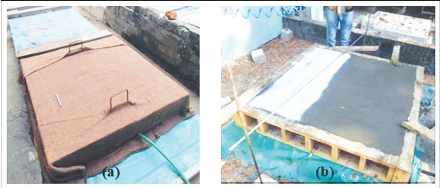
Figure 2. Curing of slabs: (a) Wet hessian curing and (b) Curing compound
